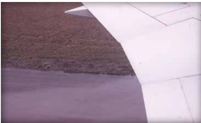
Figure 11. Airfield taxiway shoulder
