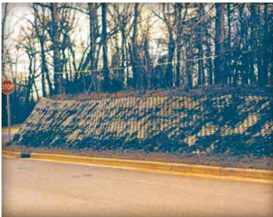
Figure 9. Embankment stabilization
