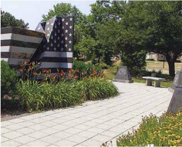
Figure 14. High SR paving slabs
